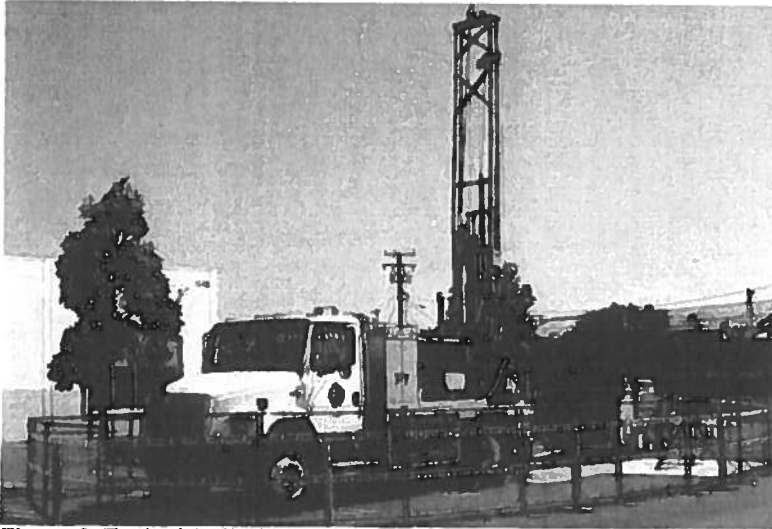
Figure 3. Typical Drill Rig Vehicle (BEI)
